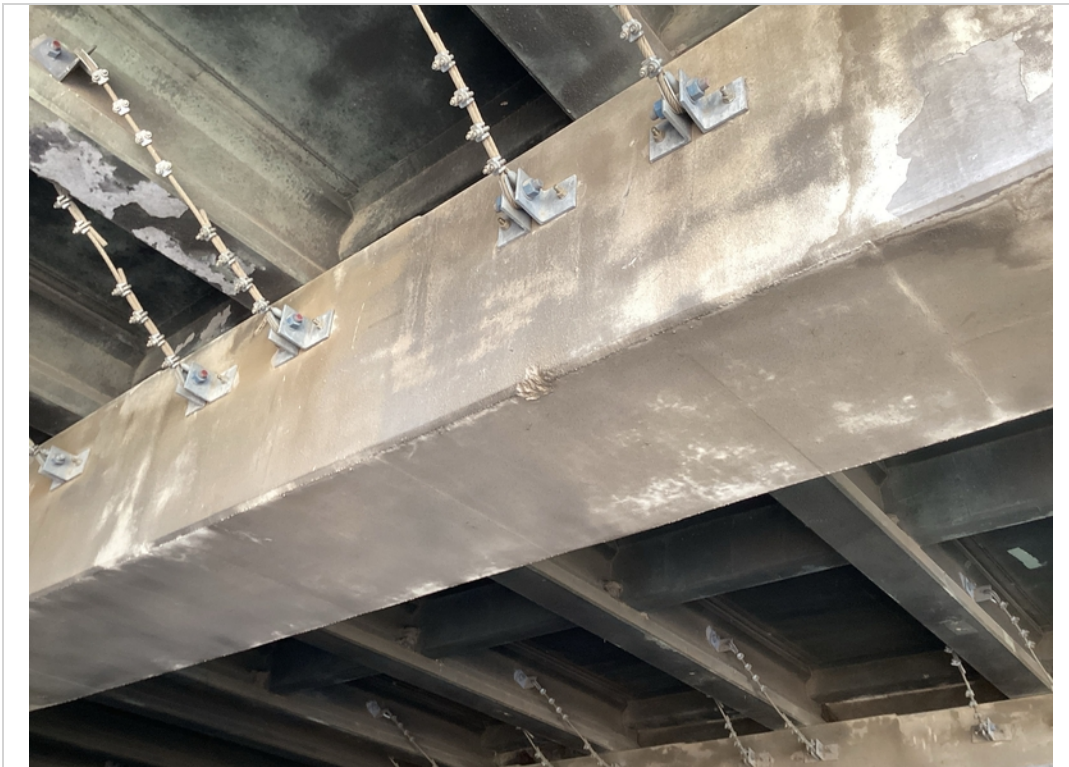
Bent 1 cap, spalling
