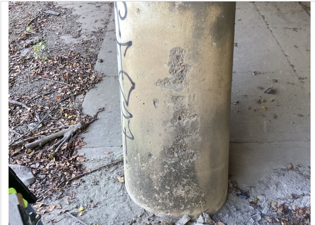
Bent 1 , Column F , collision damage
