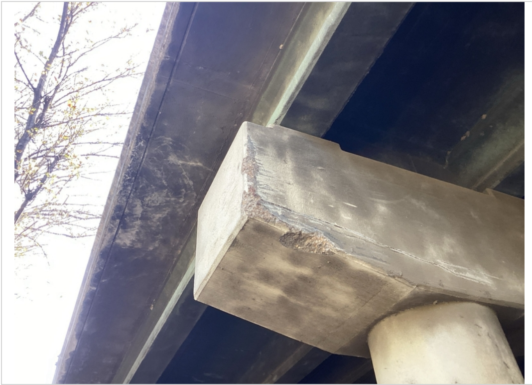
Bent 1 cap, collision damage
