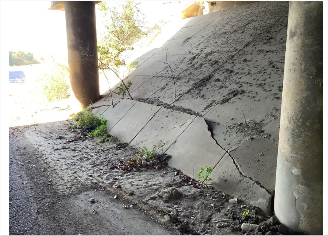
Broken area abutment 2 slope paving 18 ' wide x 6' long
