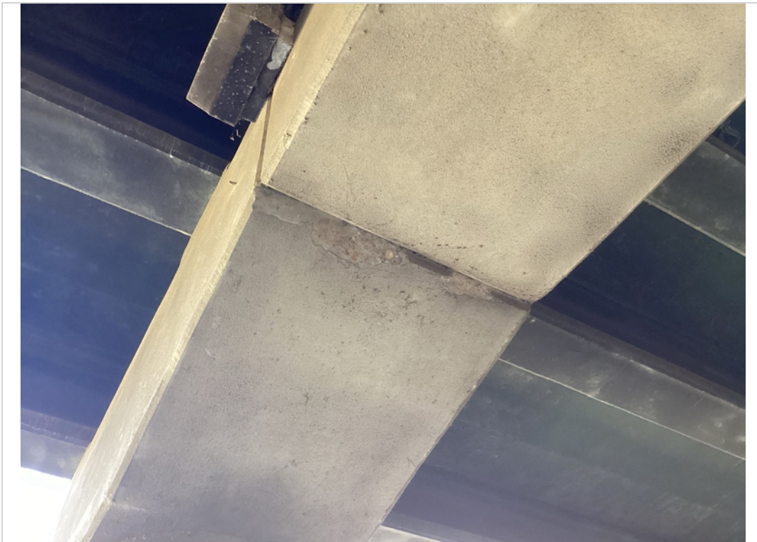
Bent 1 cap, spalling
